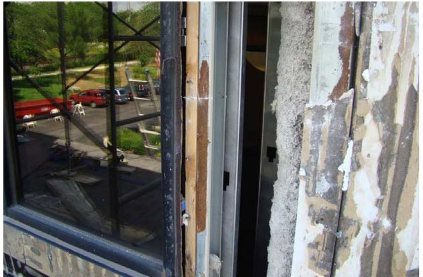
Metal studs rusting due to leakage
